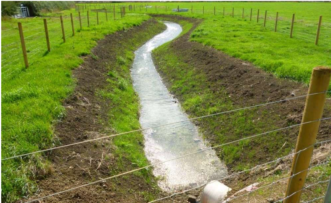
Figure 7 – Newly formed Swale
