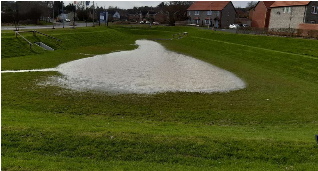
Figure 6 – Typical Detention/ infiltration basin
