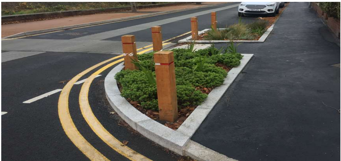
Figure 5 – Typical Bioretention System/ Rain Garden
